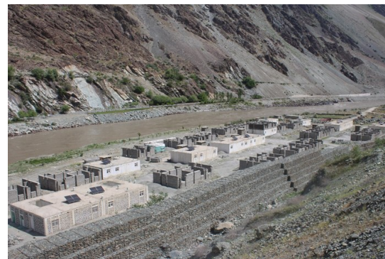
Figure 14. Structural mitigation projects, flood protection wall along Mullah Khil in Baghlan Markazi ( left ) and gabion wall as rock fall mitigation ( right ).
