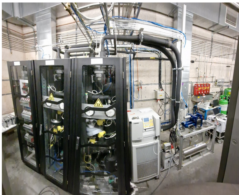
Figure 5. R134a recuperation plant installed at the CMS experiment and connected to the RPC detector gas recirculation system.
