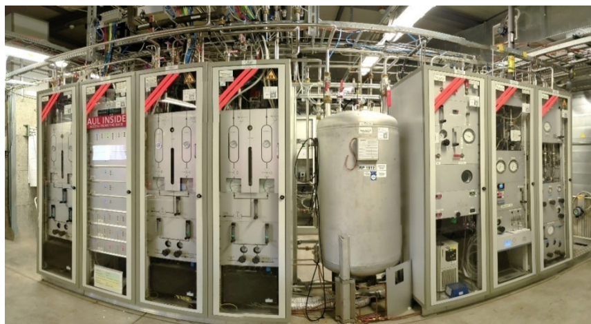
Figure 2. View of gas systems modules present in surface for one detector at the LHC experiments.
