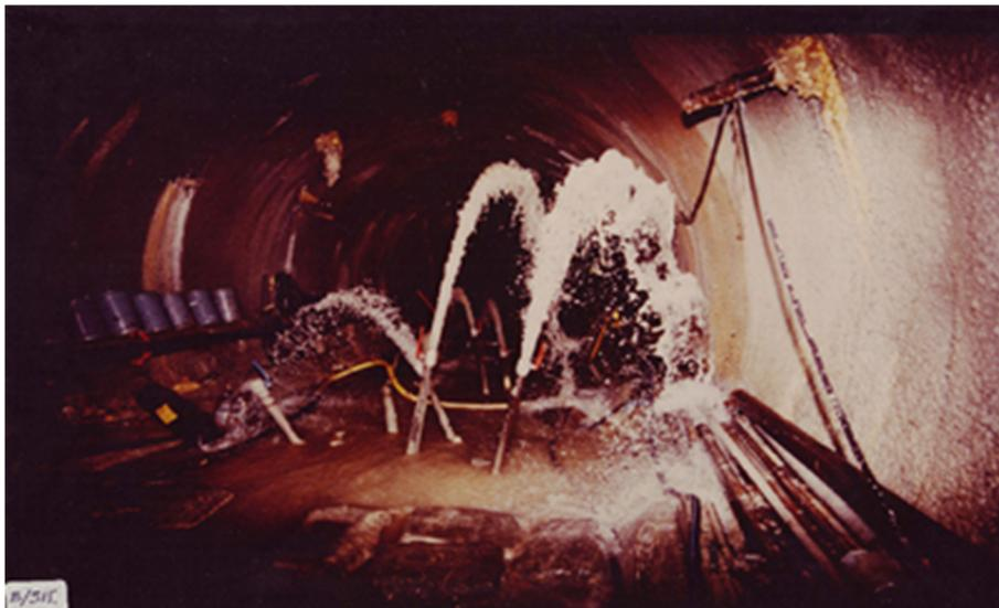
**Figure 6.** (a) Layout of the LEP ring, the 4 experiments and the LEP injectors. (b) Photo of water input to LEP tunnel.
